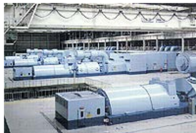
Low-loss turbine generator
