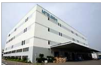
Air Conditioning and Refrigeration Systems Works
