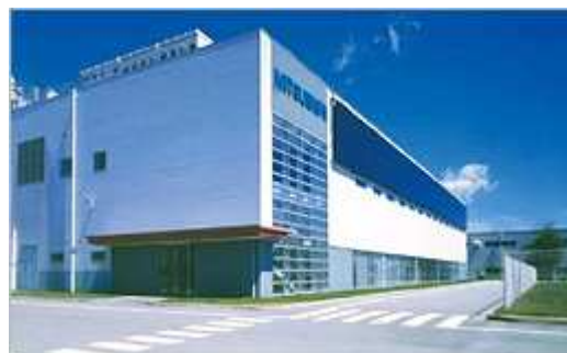
Nakatsugawa Works Iida Factory is home to our photovoltaic power generation systems business
