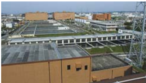
Murano Water Purification Plant
