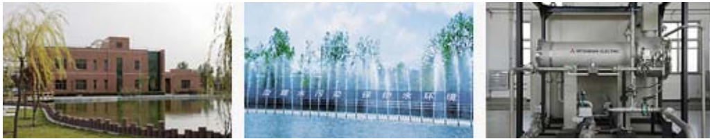
Qinghe Wastewater Treatment Plant and Mitsubishi Electric's ozone generator
