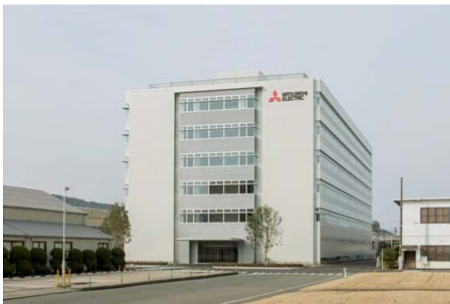
Power Device Works
