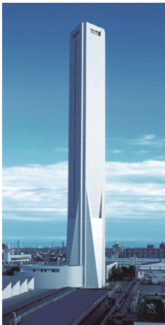
SOLAÉ elevator testing tower
