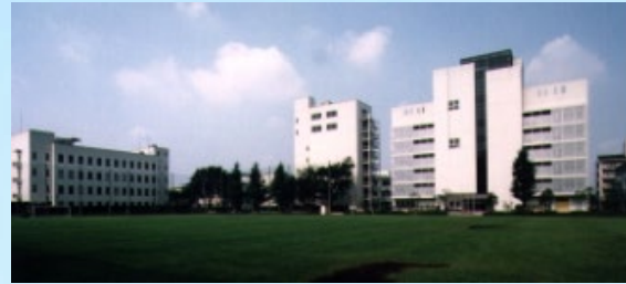
Educational Center Mitsubishi Electric Building-Techno Service
